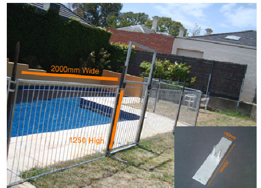
FIG.1. TEMPORARY POOL FENCE
